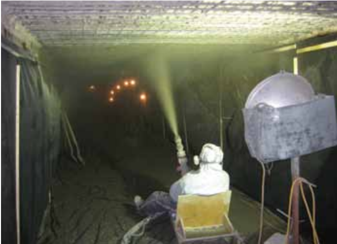
Nozzleman applies shotcrete from movable chair; Portage Bridge, Ottawa, ON, and Gatineau, QC, Canada
